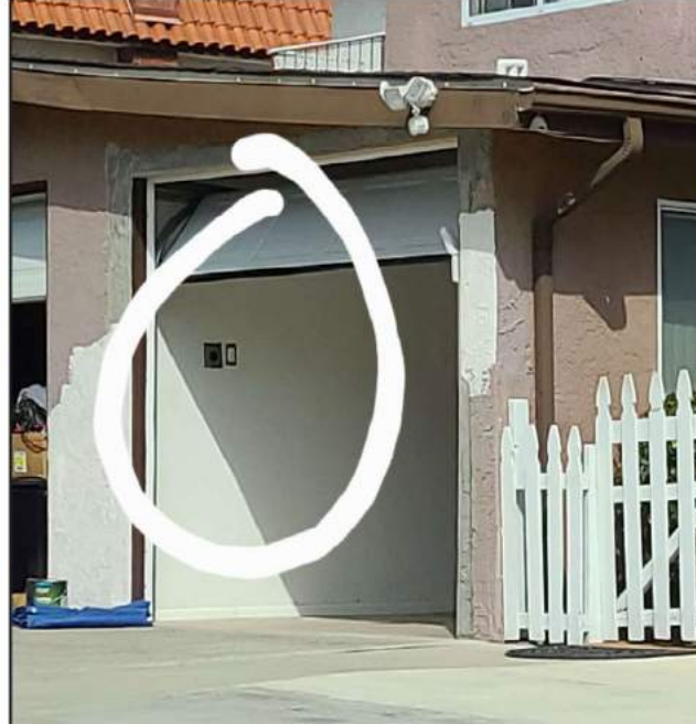
Single Car Garage after new Outlet; looks to be a 110 and 220V
