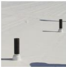
TPO Roofing System
