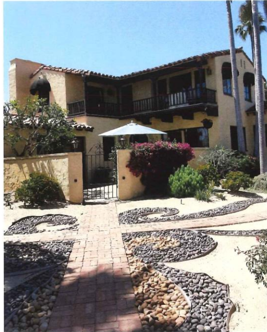
Entry looking NW
