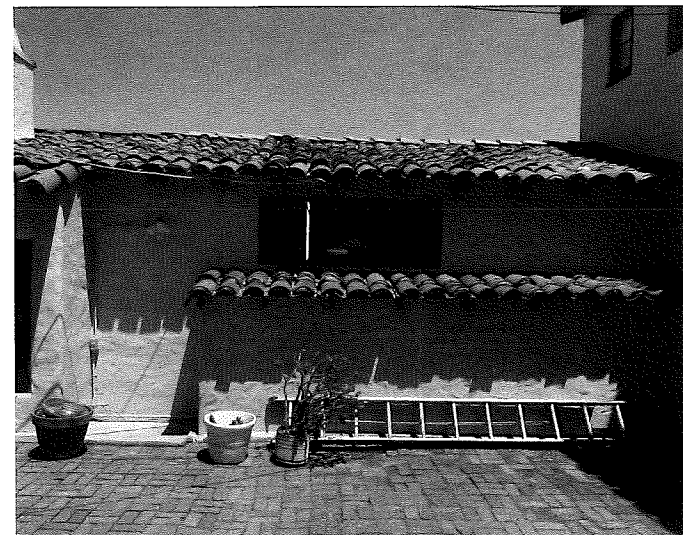
existing wall and roof tile colors
