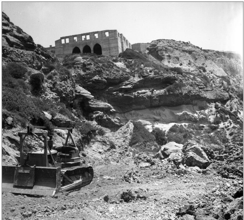
Figure 40. Partially-constructed Dana Point Inn, n.d. (Orange County Archives).
