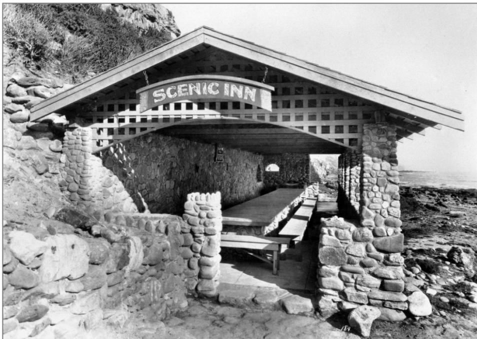
Figure 16. Scenic Inn at the foot of the bluffs, c. 1927 (Orange County Archives).
