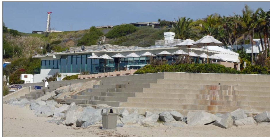
Figure 65. Monarch Bay Club, constructed in 1965 (ARG).
