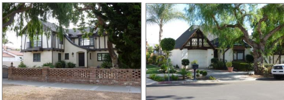
Figures 68 and 69. Examples of Tudor Revival architecture in Dana Point (ARG).
