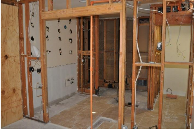
Typical bathroom renovation.
