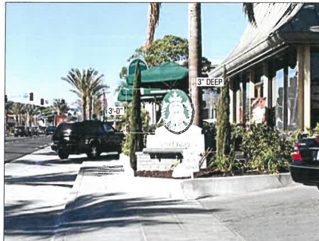
3 MONUMENT SIGN W/ DOUBLE FACE SAND-BLASTED WOOD LOGO - EXISTING CONDITION SCALE: NTS
