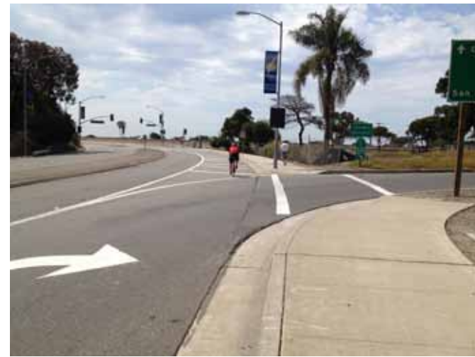
PCH Connector, Coast Highway and Doheny Park Road intersection looking southeast - Note cyclist's use of right-turn-only lane to proceed straight to Coast Highway
