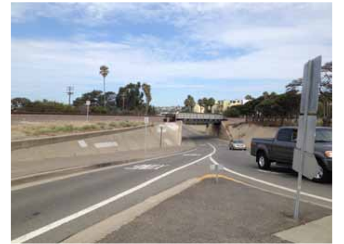
View of PCH Connector from intersection with Coast Highway and Doheny Park Road - Note uncontrolled right slip lane approaching crosswalk
