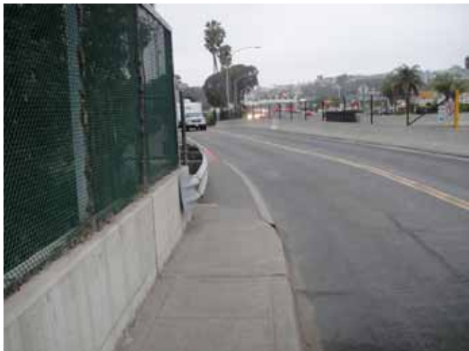
Northwest end of Park Lantern bridge over San Juan Creek - Note extremely narrow connection from Doheny State Beach pathway (red curb ramp)
