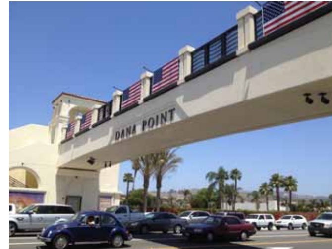
Pedestrian bridge over PCH connecting north side to Doheny State Beach
