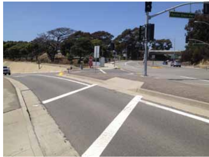
View northwest of crossing conditions at intersection of PCH Connector, Coast Highway and Doheny Park Road - Note approaching vehicle at left from PCH Connector with no traffic controls
