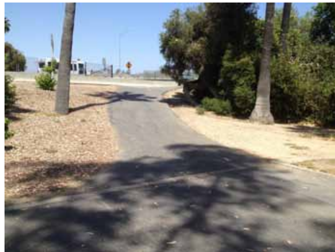
Pathway through Doheny State Beach to bridge connecting two halves of park - Note traffic on PCH Connector beyond K-rail separator in background
