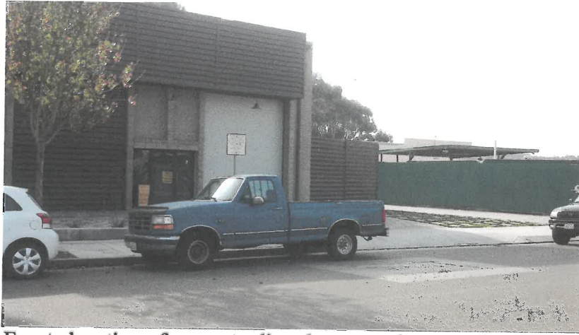
Above: Front elevation of property directly across the street of subject property
