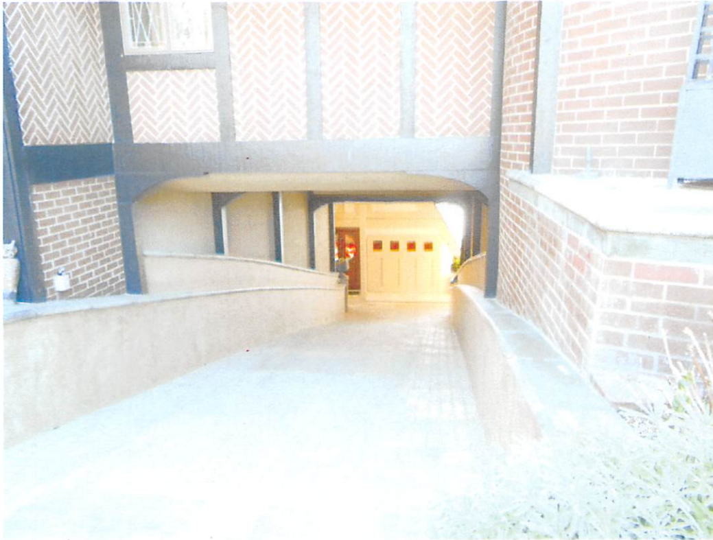
Attachment #3 – View of South Elevation of A-Frame From Tunnel
