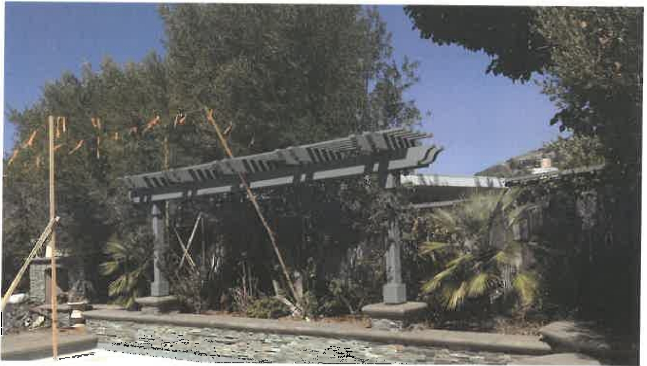
adjacent neighbor to the north - side elevation
