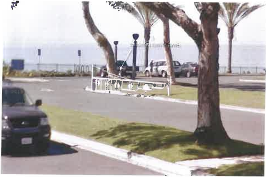
Existing Gate at Selva Parking Lot Entrance (to be removed)
