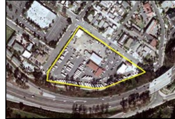
Site 3: Capistrano Unified School District Storage Yard
