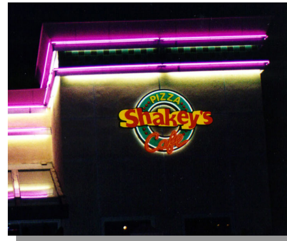
The use of neon tubing can add nighttime interest to a building but should be carefully used and in limited amounts.
